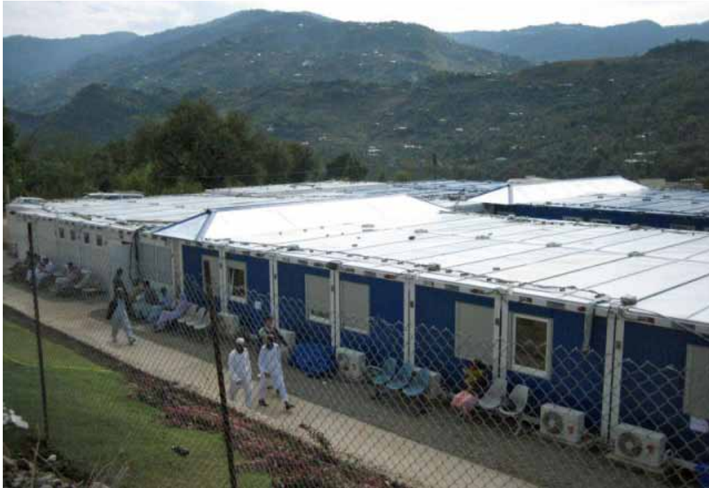
CONTAINER HOSPITAL BAGH MSF, PAKISTAN
