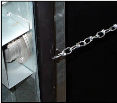
28. Attach chain to hook as shown.
