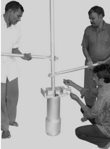
Lifting spanner in operation
